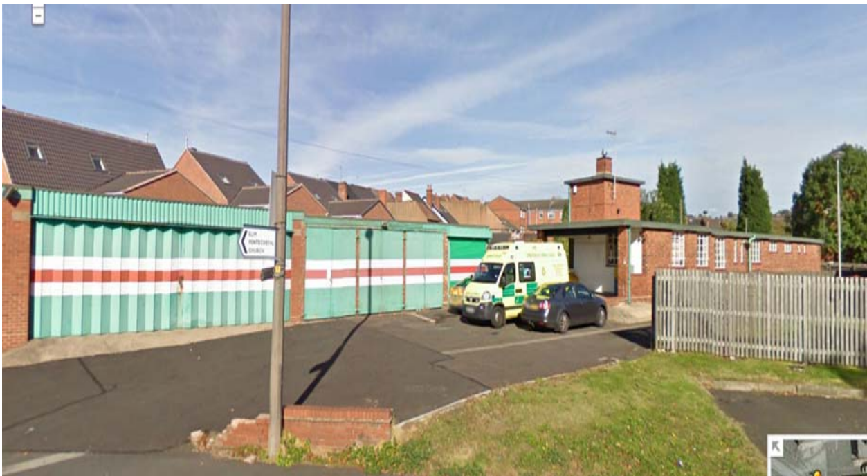
Street View of Cradley Heath Ambulance Station off Lawrence Lane
